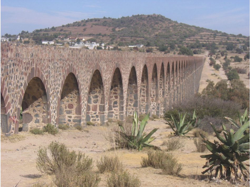
Figure 1. The aqueduct at Otumba, Hidalgo, México built in the 1540s, purportedly under the direction of Fray Francisco de Tembleque (Valdes 1961)
