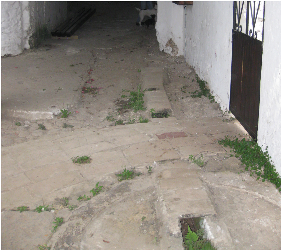
Figure 8. The mill chase at Hacienda de Pacho through which the turbines could be accessed. Water flowed out of the mill through the covered canal in the lower right.
