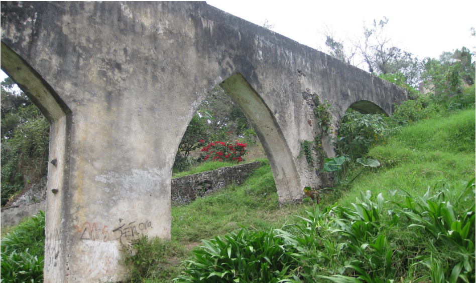
Figure 6. In addition to having a circular arch (right) this aqueduct is characterized by Gothic arches.
