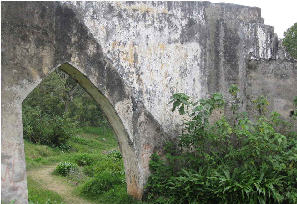
Figure 7. A view opposite that of Figure 6. Clearly evident are the widened pier/narrowed span, and the addition of a penstock.
