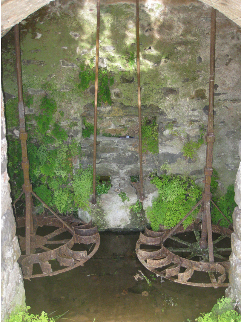
Figure 16. The two horizontal turbines turned by water falling through the penstock.
